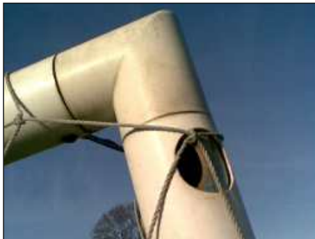
Figure 26 Samba goal with net supports spragged in holes with no proper roof to net.
