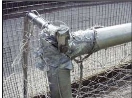
Figure 35 Badly designed goals have been damage by the aid of poor maintenance (not an ITSA goal product).
