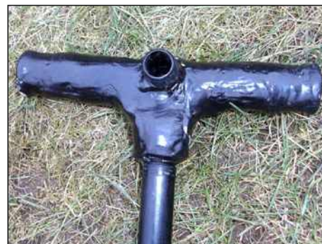
Figure 4 Broken pump needed repair not long after purchase
