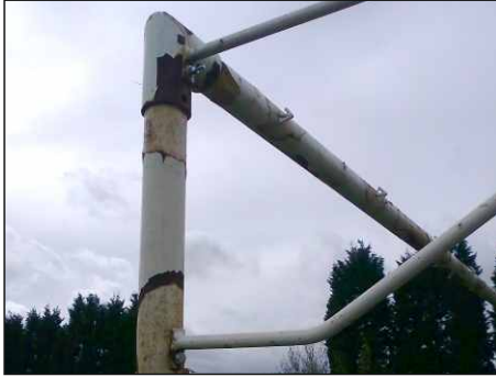
Figure 44 A typical local authority football goal with bolts missing - can not line up & can not be secure (not an ITSA goal product).
