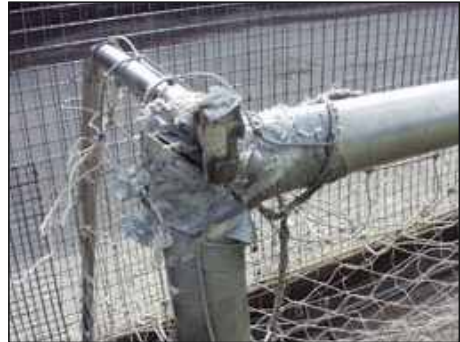
Figure 35 Badly designed goals have been damaged by the aid of poor maintenance (not an ITSA goal product).
